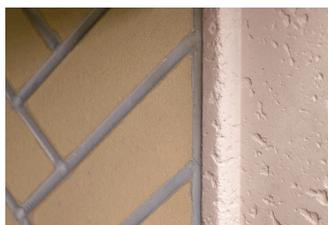
A flush-hearth design enables a seamless transition from firebox to finishing materials.
